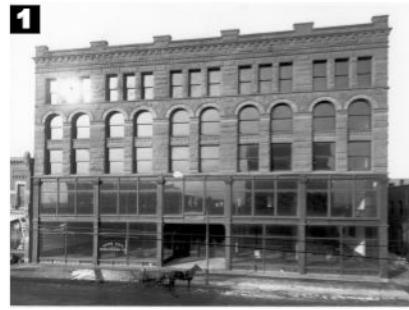
Northwest side of the street
